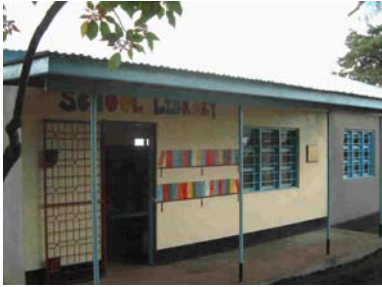
A new library building at Masia primary school
