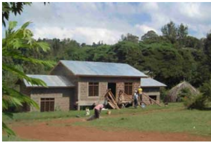
The new Village Crafts shop and Chagga house
