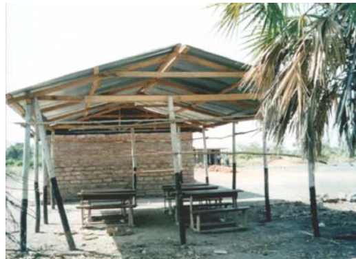
Kochakindo's new shelter is an improvement at least
