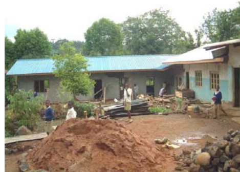
Kilaremo primary school undergoing renovation
